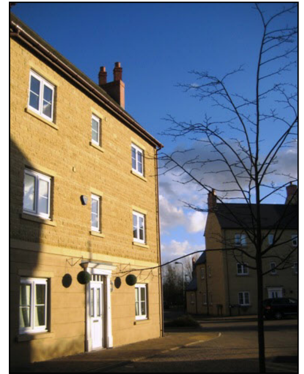
Interior of St Mary's (top) and new housing near Bridge Street (above)
